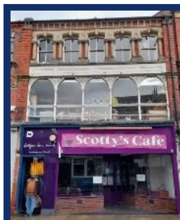
Figure 46 17 Cross Street before the work began. Samantha Jones.
