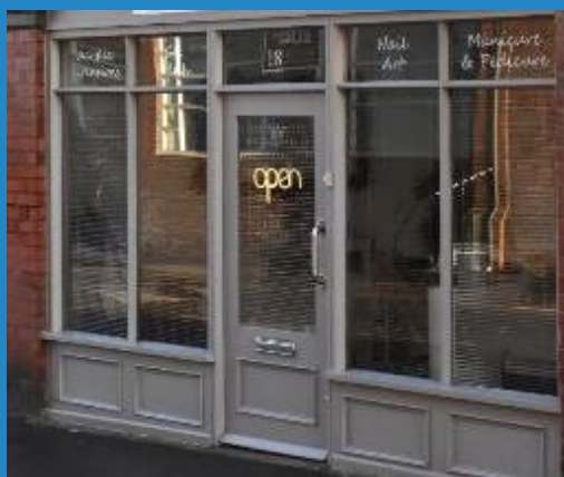
Figure 18 Windows clear of stickers and signs are most appropriate for traditional shopfronts. This property on English Walls uses stick on lettering in the upper panes to good effect.
