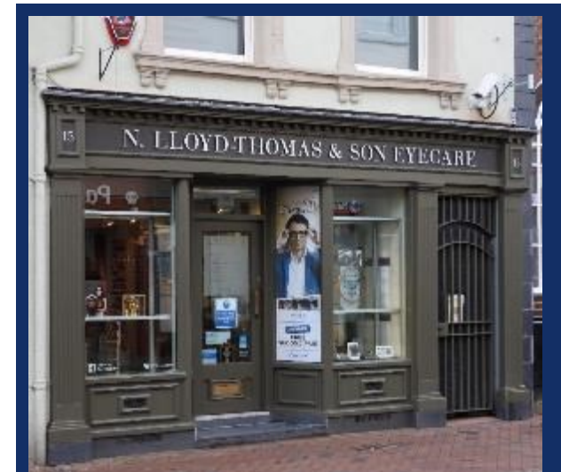
Figure 45 This restored shopfront on Church Street uses traditional materials including a hard wood timber fascia and stallriser on a stone plinth. Henry Thomas.
