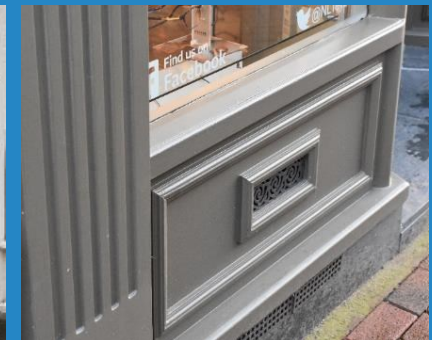
Figure 37 Metal grilles are both practical and decorative. They have been effectively incorporated into this modern shopfront on Church Street.
