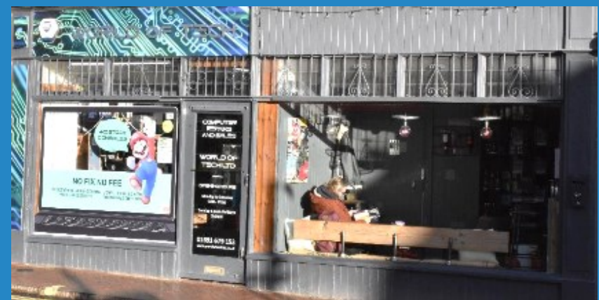
Figure 20 Contrast the clear window of the cafe on the right with the abundance of stickers to the door and shop window of the left hand property. These detract from the traditional shopfront and the overall appearance is less visually appealing. Leg Street.
