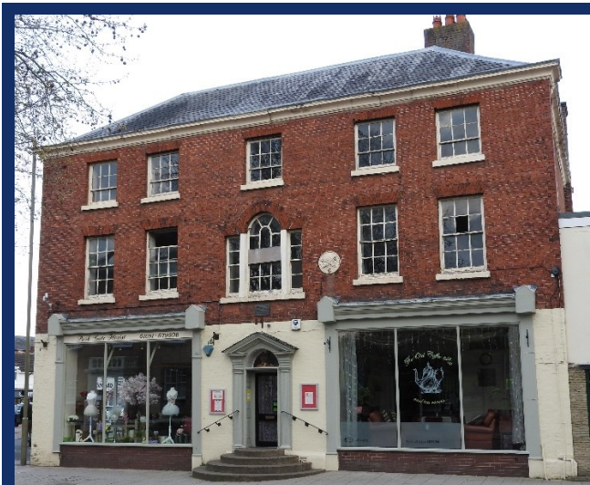
Figure 10 Although the two shopfronts of this building on Church Street have been altered and simplified over time, they retain the harmony and balance of the early 19 th century building as a whole. Credit: Henry Thomas.
