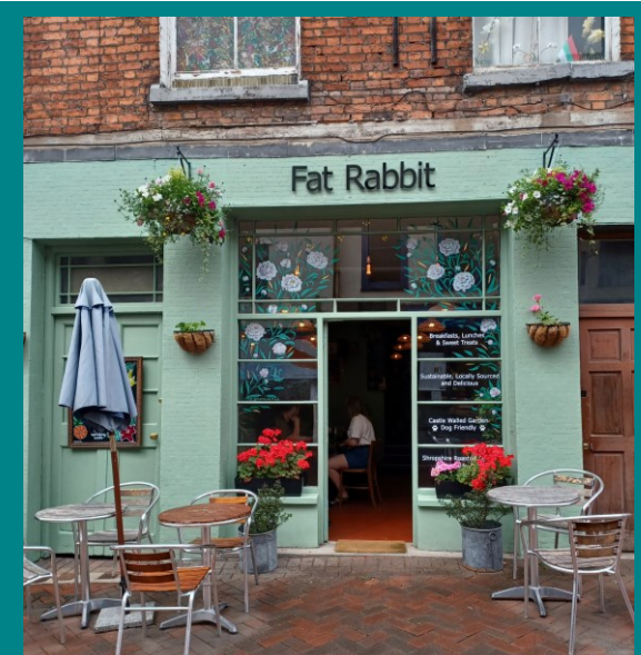
Figure 17 This café on Bailey Street retains the 20 th century glazing but has a contemporary colour scheme and sign. Importantly, the contemporary features including the window art and colour scheme are reversible interventions. Samantha Jones.
