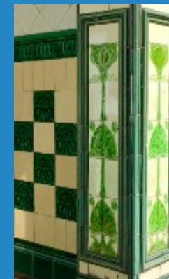
Figure 33 Glazed tile pilaster, Leg Street. Richard Banks.
