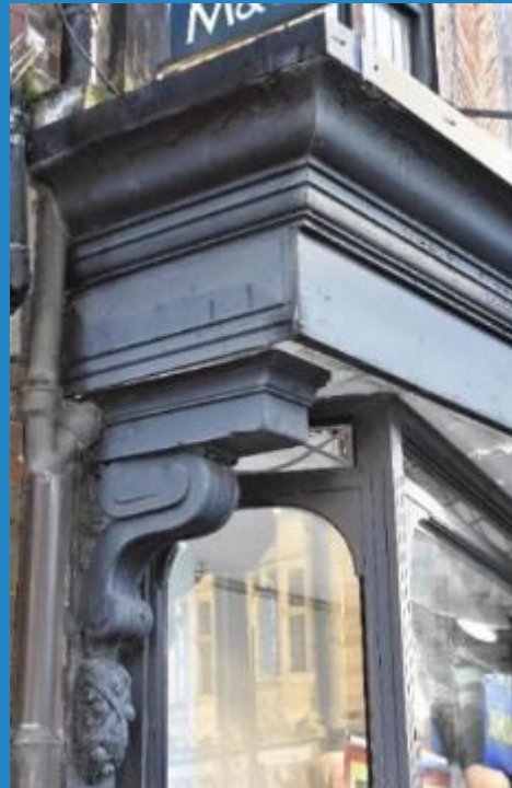
Figure 27 A deep cornice with chamfered mouldings, The Cross.
