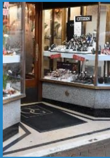
Figure 22 Attractive recessed entrance. Church Street.
