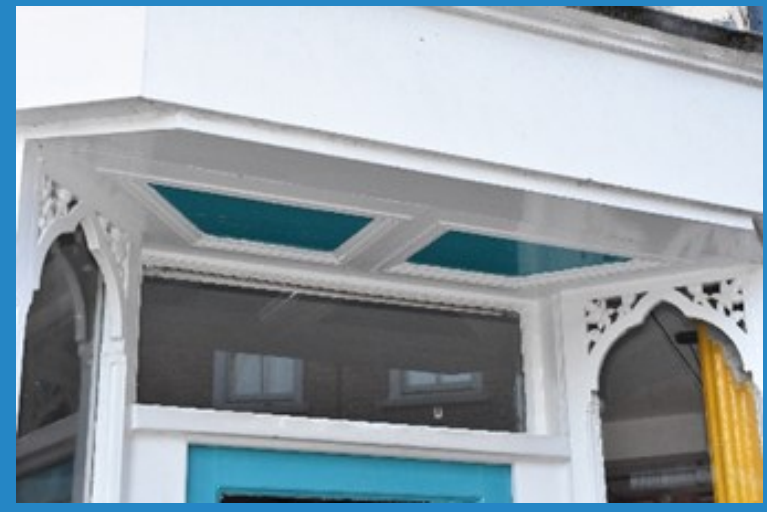
Figure 24 Recessed doorways are part of the character of traditional shopfronts. Details such as door panelling, mouldings and letterboxes can be retained and enhanced, as can tiled or decorative stallrisers.
