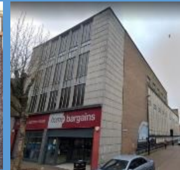
Figure 5 This superstore on Bailey Street was purpose built as Woolworths in the 1970s.
