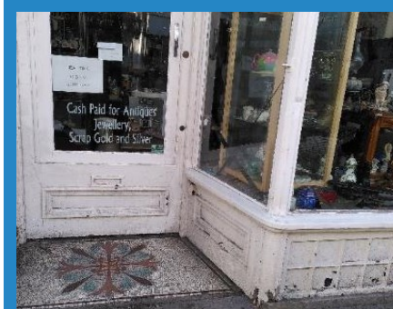
Figure 35 Early 20th century panelled stallriser on Leg Street.
