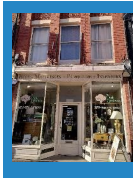
Figure 25 Mullions provide visual continuity with the upper storey windows to this property on Bailey Street.
